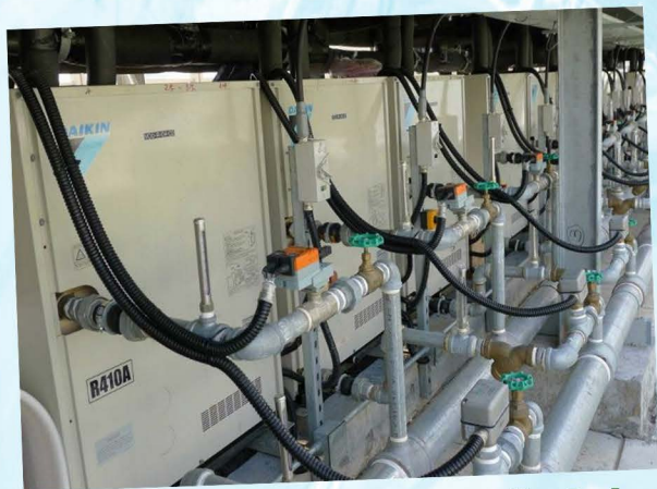
Centralized Water Cooled Air Conditioning System
